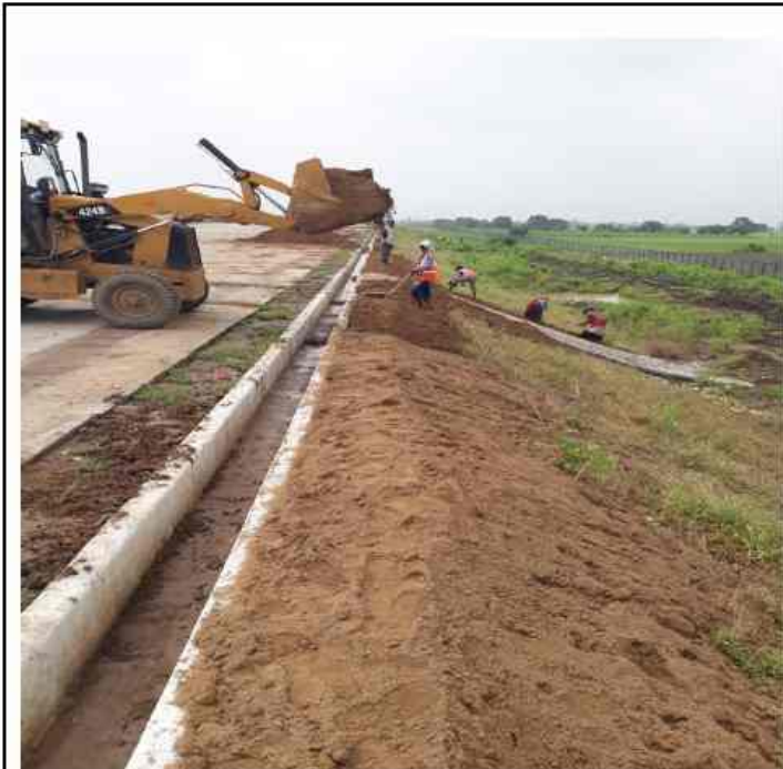
CH 312+000 Drain protection work in progress
