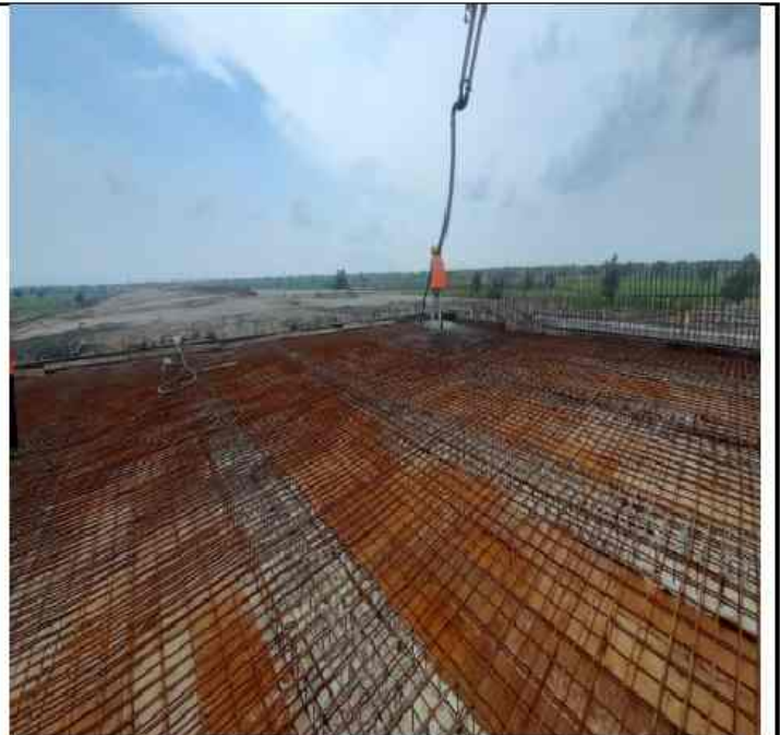
CH 309+840 MNB Deck slab pouring work in progress RHS
